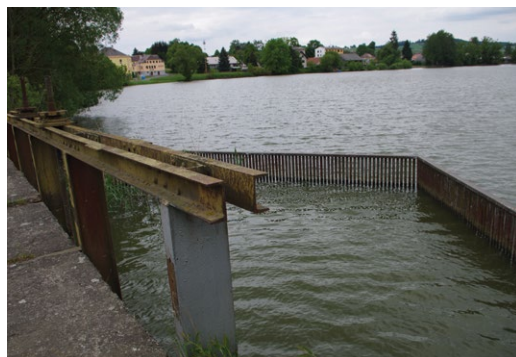
Picture 36: A screen wall in front of a safety spillway.
