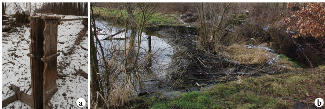
Picture 34: A monk damaged by beavers (a), a beaver dam on a security spillway (b).
