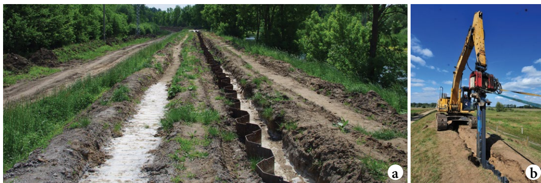
Picture 31: Steel sheet piles in a body of a flood dam (a), plastic sheet piles are driven into the ground (b).
