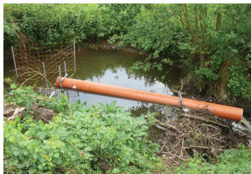
Picture 19: Improperly made drainage of a dam - the pipe after the installation was not covered (i.e. the dam was not finished), and moreover, water falls from height behind the dam, causing unwanted noise.
