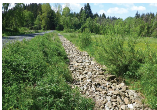
Picture 21: A road ditch filled with coarse-grained material, before there was an intermittent watercourse where beavers built dams and surge water, which endangered the road.
