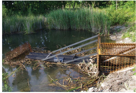
Picture 25: A culvert protection, using a hanging indent steel cage on the inflow. Two plastic pipes pulled high above the culvert inflow ensure the flow rate. Their inflow is also protected by a protective wire cage.
