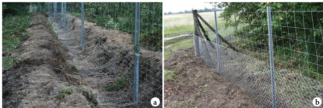
Picture 6: Fencing of a cover with a mesh, which is embedded into the ground and bent into an L-shape before the horizontal part is covered with the soil (a); an existing fence is strengthened with a new mesh (b).
