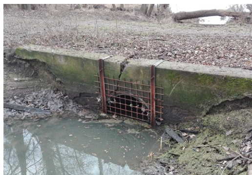
Picture 26: Improper protection of a culvert – the grill can be quickly blocked and the stability of the culvert and the road could be endangered. This solution is very risky by itself, even if there are no beavers in the location.
