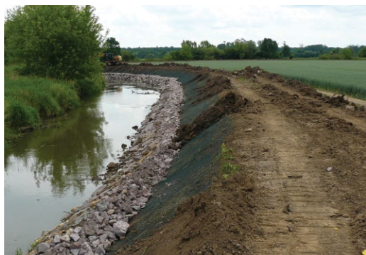
Picture 30: Placing the mesh fencing into the body of the flood dam on the Kyjovka River - the slopes are protected with the mesh fencing against burrowing, the riverbed is protected with the coarse rock-fill against the bank erosion.
