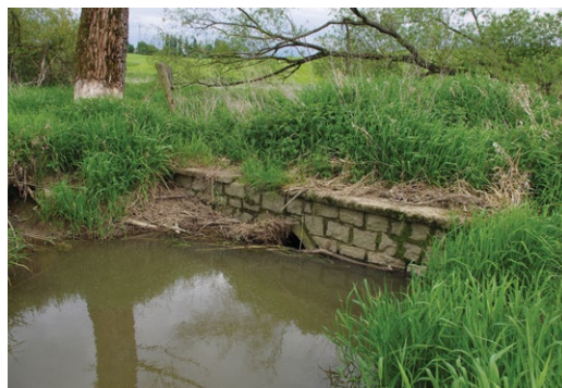
Picture 24: Partially clogged culvert by unwanted beaver activities.
