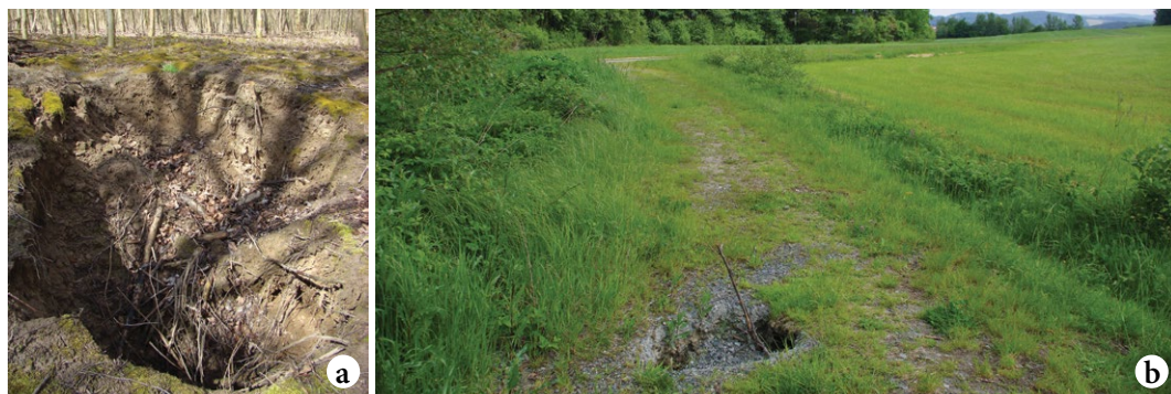
Picture 32: A fallen through burrow in a watercourse bank (a), a fallen through path (b).
