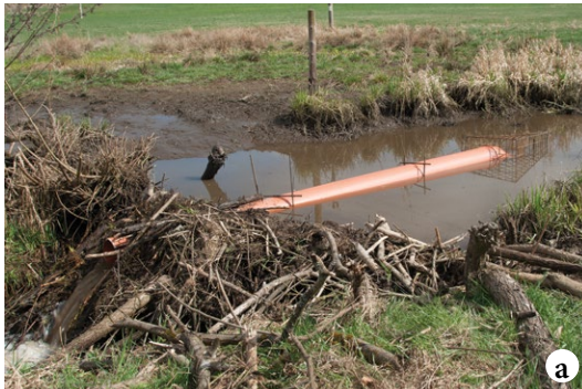
Picture 18: Drainage of a beaver dam: into a dam inserted pipe with a knee in an inflow and with a protective cage (a); detailed inflow of the pipe and protective cage (b).
